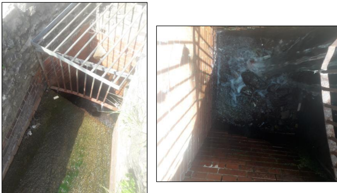
Figure 12: Image of 'Culvert Inlet 1' captured post event during CCTV surveying operations (30/07/2020) (left) and evidence of debris accumulation within the culvert chamber (right)
