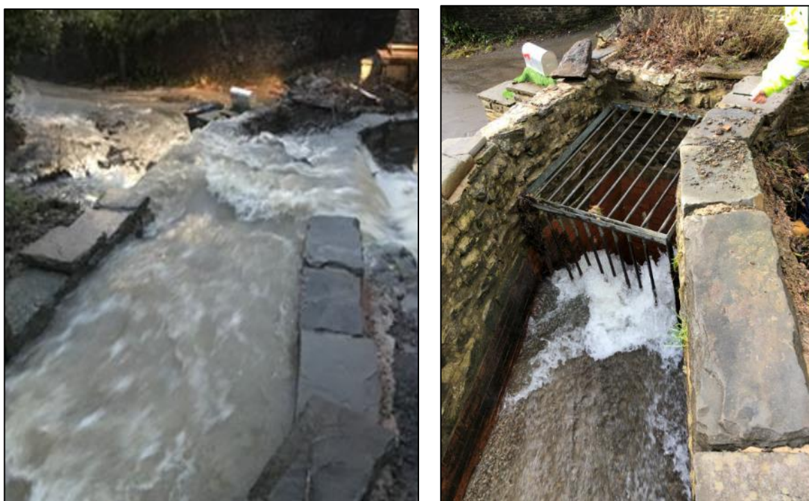
Figure 5: Evidence of 'Culvert Inlet 1' surcharging during the storm event and conveying southwards towards Column and Dumfries Streets (left) (image provided by resident), and 'Culvert Inlet 1' post storm event (right) (captured by RCT's Flood Risk Management team on 20 th February 2020)
