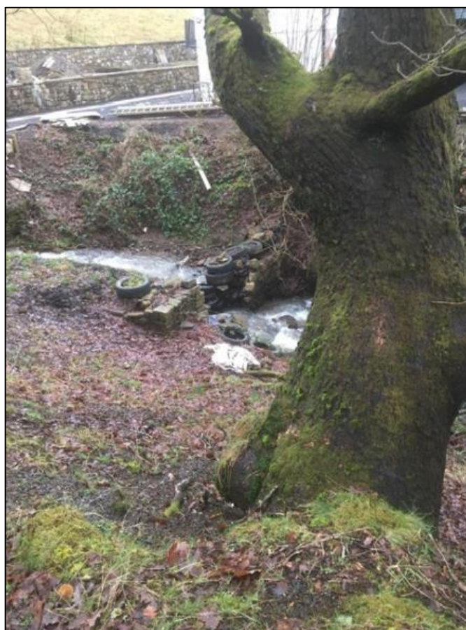
Figure 20: Image of tyre damn acting as an obstruction to the watercourse upstream of 'Culvert Inlet 2' (captured by RCT's Flood Risk Management team on 17th February 2020)
