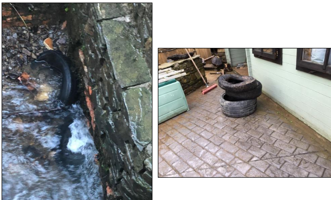
Figure 14: Evidence of debris, inclusive of tyres, causing a blockage to 'Culvert Inlet 2' during Storm Dennis (left) and evidence of the three tyres removed from the inlet by a resident (right) (images provided by resident)
