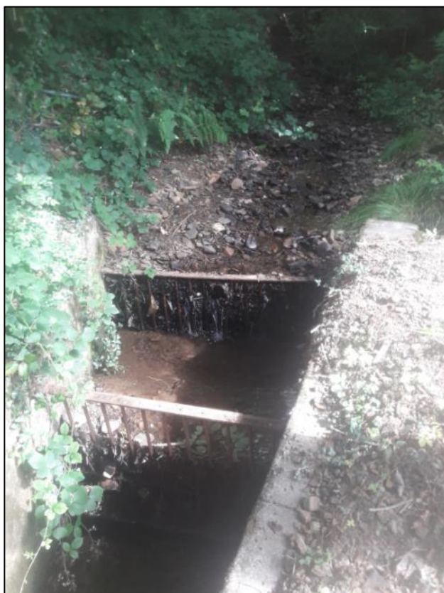
Figure 23: Photo of significant debris accumulation behind the upstream debris screens above 'Culvert Inlet 3' in the Nant Tyle-du watercourse (captured by a Council appointed contractor on 03/08/2020 during CCTV survey operations)
