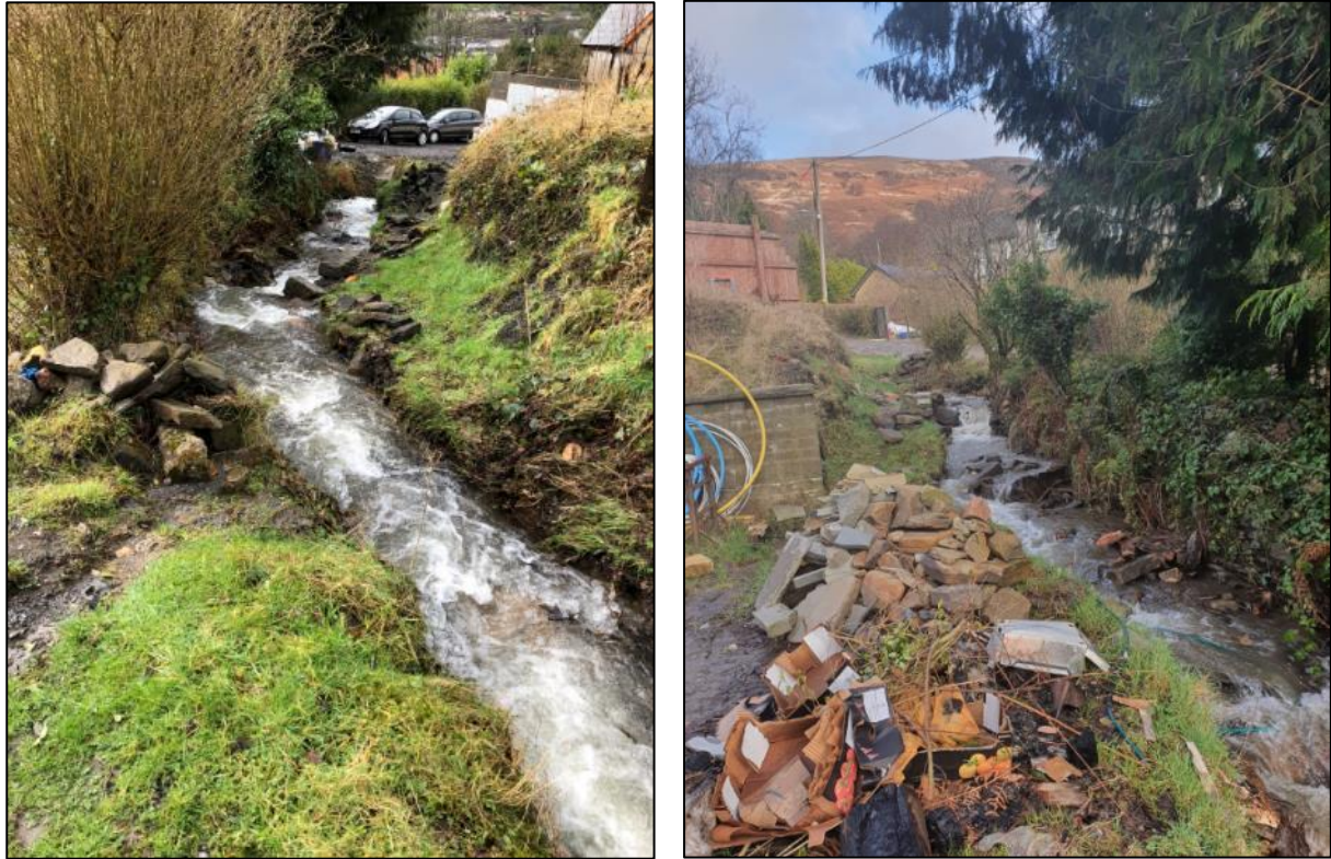
Figure 22: Unnamed open watercourse upstream of 'Culvert Inlet 1' showing evidence of large stones within the channel and surrounding embankment area (captured by RCT's Flood Risk Management team on 20 th February 2020). Looking downstream towards 'Culvert Inlet 1' (left) and looking upstream towards the outfall of 'Culvert Inlet 2' (right).
